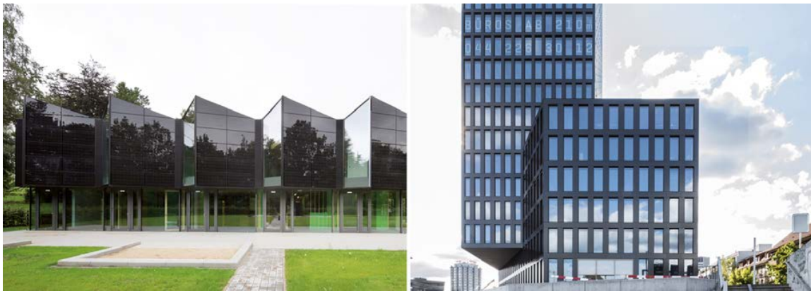
Fig. 18/19: Nursery +e, Marburg (2014), opus Architekten (left) and Grosspeter Tower, Basel (2017), Burckhardt+Partner (right)
