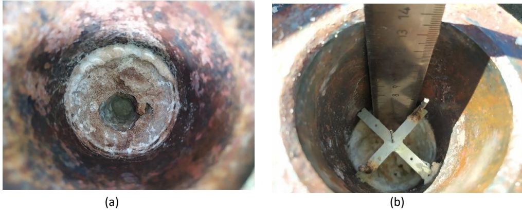
Fig. 7. Finned cylinder inspection after the second melting/solidifying cycle with increased salt content. (a) Non-uniform salt block, (b) Empty height showing the thermocouple brackets.
