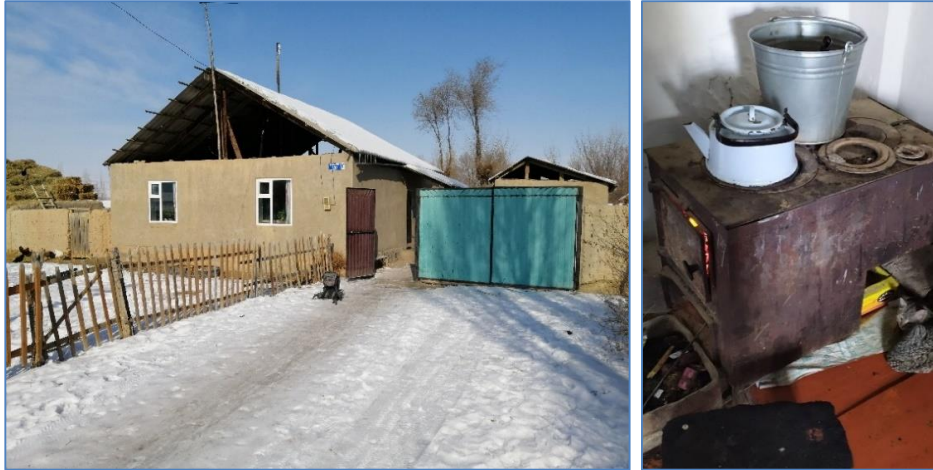
Fig. 1: Typical rural residential house in Kyrgyzstan with an open-roof construction (left) as well as a traditional heating stove (right) which is used for cooking and heating up one or two rooms of the building
