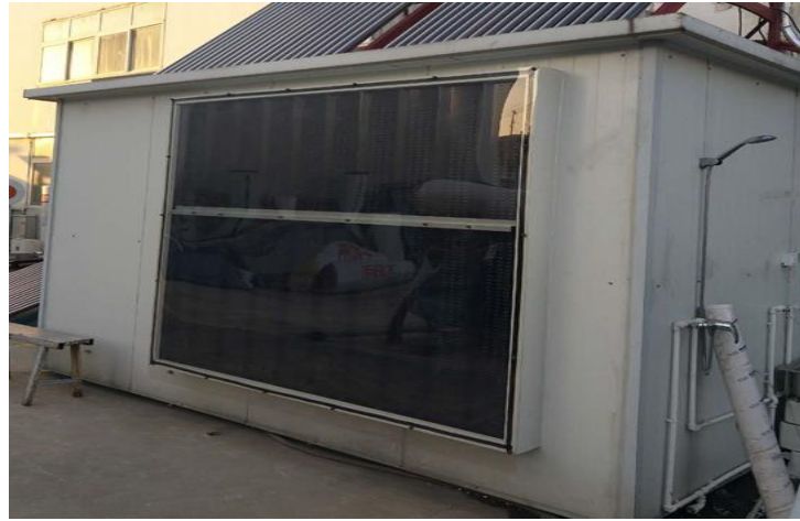
Fig. 6: Space heating system
