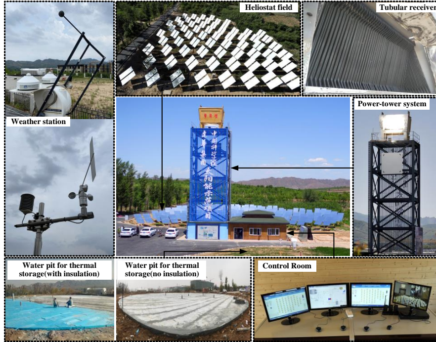
Fig. 3: The long-term water pit thermal storage/heating system in Huangdicheng town
