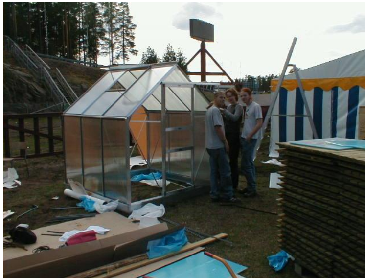
Fig.1 A set up to demonstrate greenhouse effect being built at Teknoland. Exhibit label: A higher temperature can be experienced inside the greenhouse (as compared to temperature outdoors) demonstrating the greenhouse effect.
