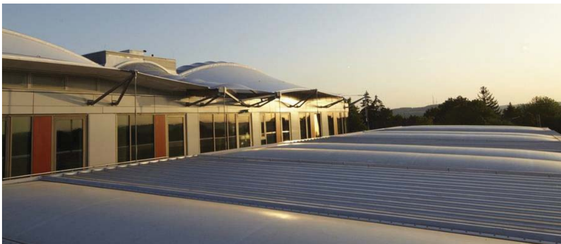
Fig.1: Energy Efficiency Center viewed from north-east, the north-orientated rooms on the first floor and the roof of the technical center. Clearly visible is the textile roof with translucent PTFE-glass membranes and partially transparent ETFE films in the ridge of the roof.
