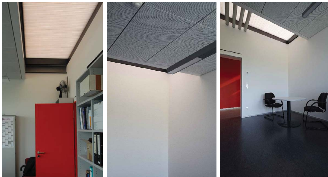
Fig.2: Aerogel glazing in the back of the offices
