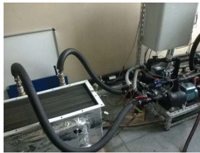
Figure 5: detail of the storage during tests.
