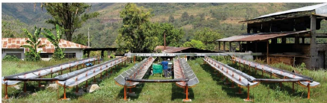
Fig 3: Picture of 60 linear parabolic concentrators in AGROINKA tea factory.
