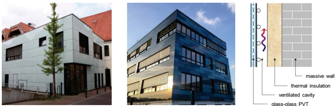
Fig. 1: Examples of ventilated glass façades with common glass panels (left, source: Konvortec) and PV panels (center, source: Konvortec) as well as schematic representation of the ventilated façade with glass-glass PVT panels under development (right)
