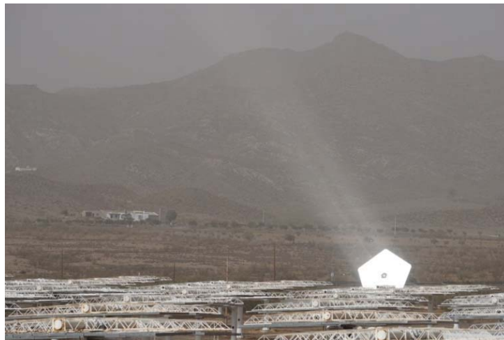
Fig. 2: This figure shows the low visibility and the light scattered by the large particles in the atmosphere on 22 nd February 2016 at 14:30 in PSA. Solar radiation reflected by the heliostats is attenuated by scattering.
