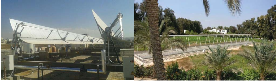
Figure 3. PTC at Irbid, Jordan (left) and LFR at Egypt Markaz Belbes (right)
