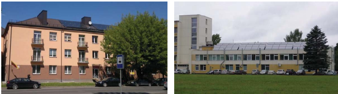
Fig. 1: The first solar thermal system 60 m 2 in multi-family building in Panevėžys city and the biggest solar thermal system 204 m 2 in Plungė town hospital (till the end of 2015).
