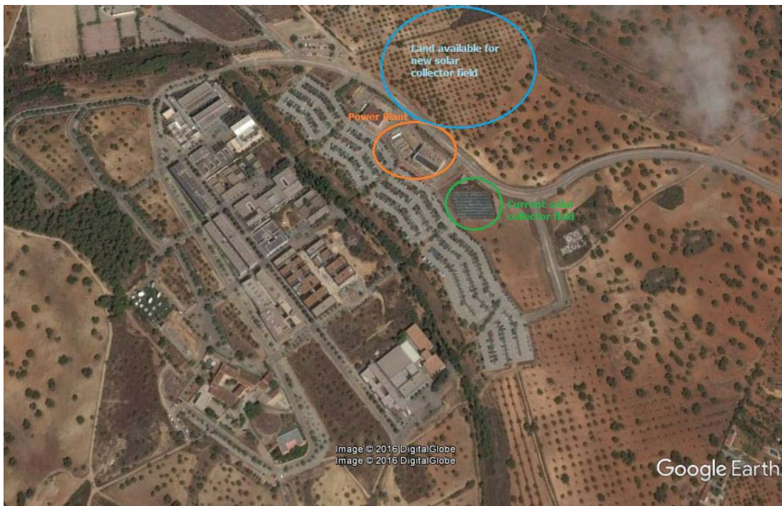
Fig. 2: New solar system location.
