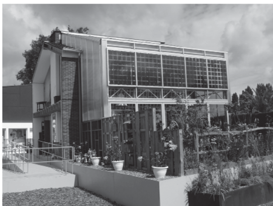
Fig. 8: The TU Delft entry to the competition in Versailles was the retrofit of a typical Dutch terrace home. Source: University Wuppertal
