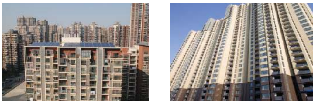
Fig. 2: View of real projects using these two installation types for solar collectors
