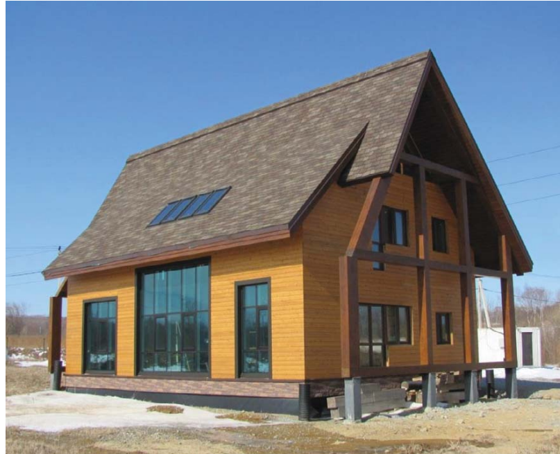
Fig. 4: General view of the house from the south-east in the winter of 2015-2016
