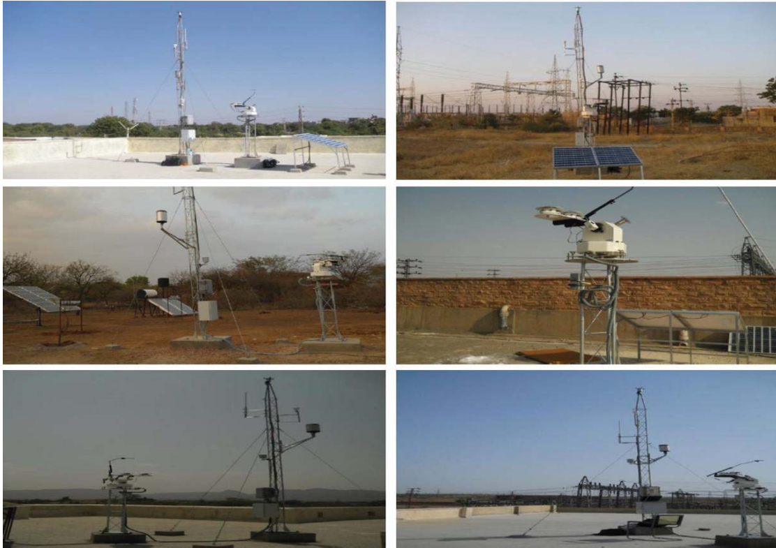
Fig.2: SRRA stations at Bagora (top left), at Balotra (top right), at Kota (middle left), at Mathania (middle right), at Ajmer (bottom left) & at Phalodi (bottom right).
