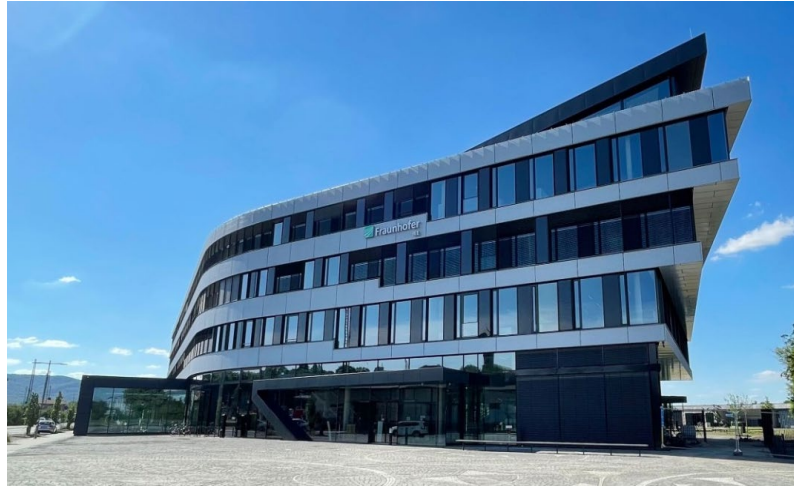
Fig. 6: New institute building of the Fraunhofer IEE in Kassel
