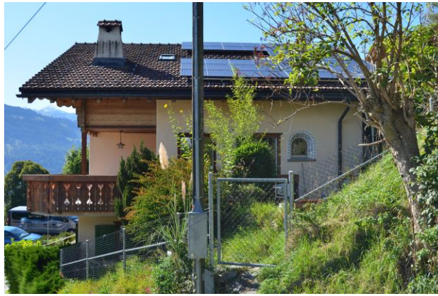
Figure 3: Pilot building in Pany (GR), Switzerland.
