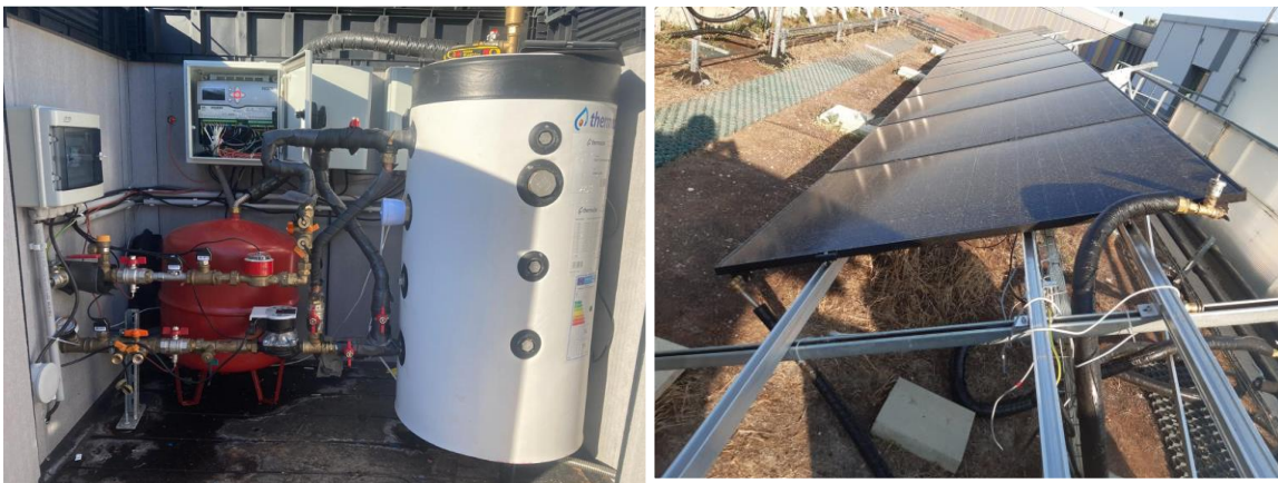
Fig. 1: (a) Photo of the test bench technical room (b) Photo of the row of PVT panels on the flat roof
