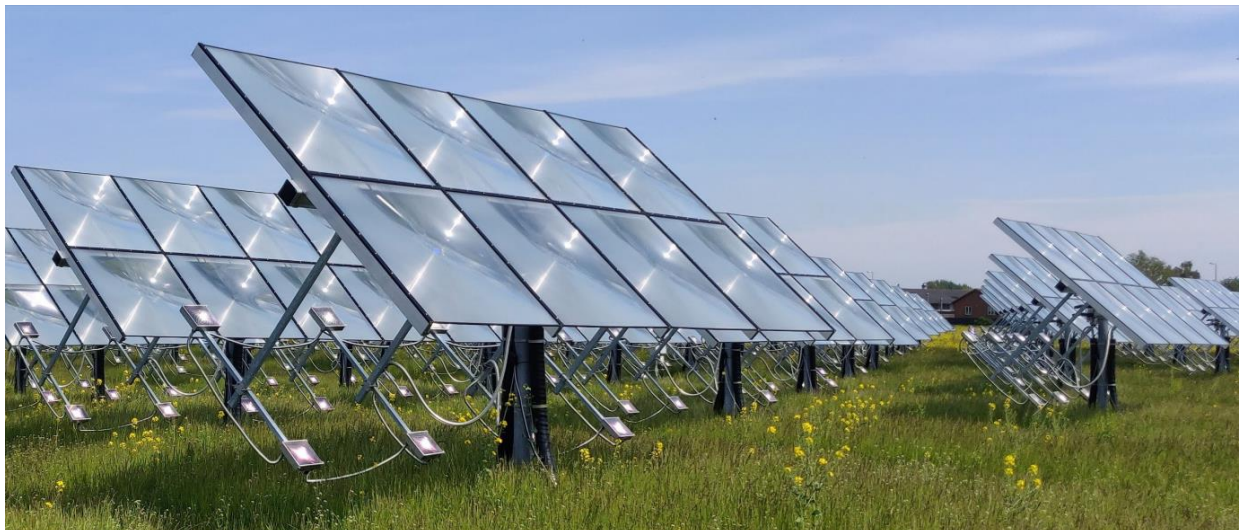
Figure 6 Photo of Fresnel lenses, Heliac in Denmark (Jensen et al. 2022)
