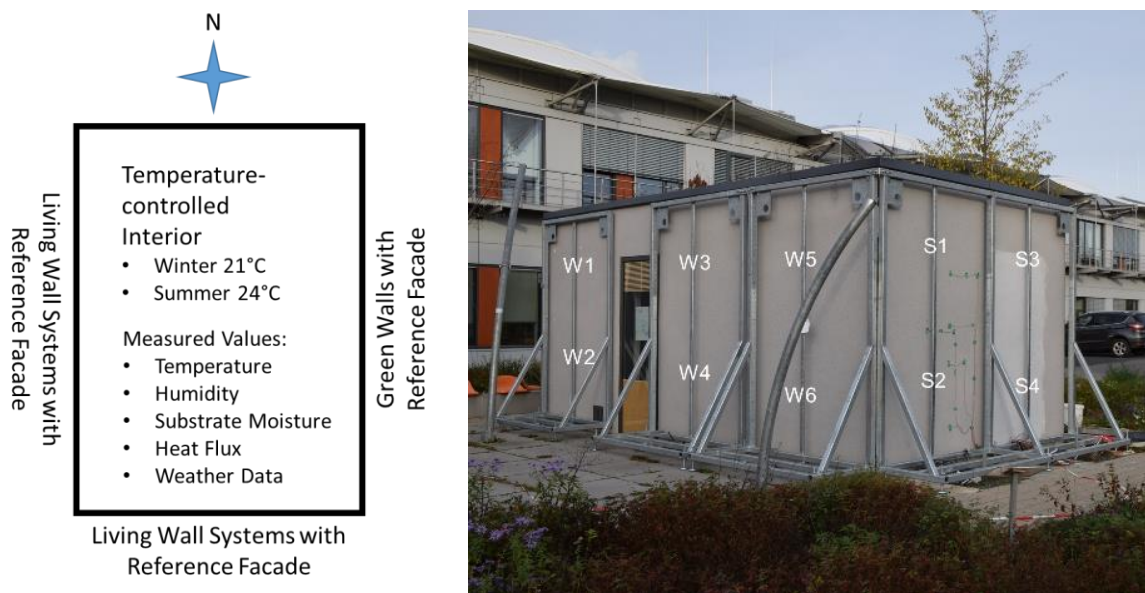
Fig. 2: Sketch of the measurement setup for LWS on our outdoor test facility (left) and southwest view of the test facility with frames for the LWS and designations for the wall sections (right).
