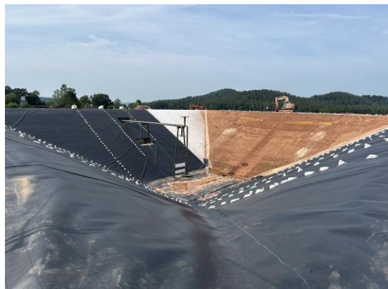
Figure 5: Construction progress of the PTES (image as of July 2024).
