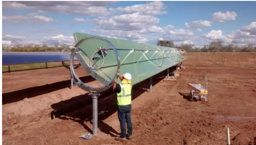
Figure 22. 175 kWth solar waste management system in City of Surprise, AZ (Image Credit: Rackam)
