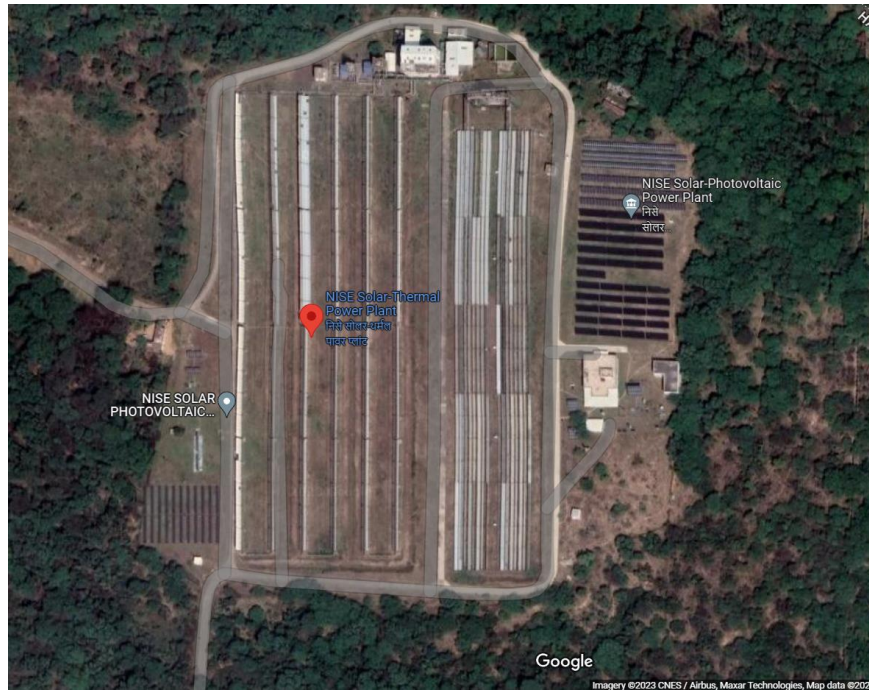
Fig. 1: Satellite image of the power plant located at Gwalpahari (Google Maps, (2023))
