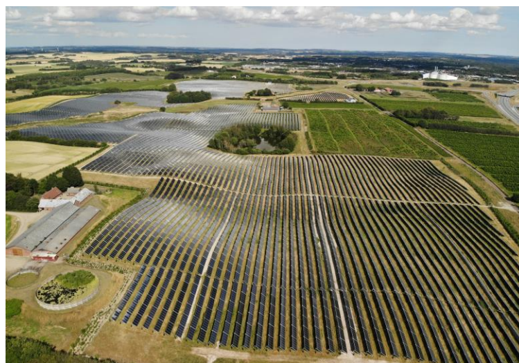
Fig. 1: Solar district heating plant in Silkeborg (156,694 m 2 )
