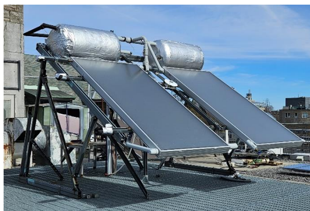
Fig. 2: Installation of identical thermosyphon domestic hot water heaters installed for testing.
