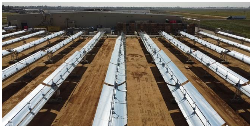
Figure 11. 2.3 MWth solar steam facility for almond pasteurization in Madera, CA [(Epp, 2022), Image credit: Sunvapor]
