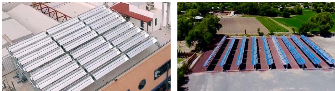
Figure 1212. a) Absolicon's rooftop PTC for IPH application in Greece (RTC, 2023); b) Inventive Power's ground mount application in Mexico (Rosell, 2022). Image Credits: Absolicon and Inventive Power
