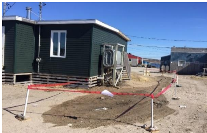
(b) Heating oil leak from storage tank (Photo taken by Edua Jones)
