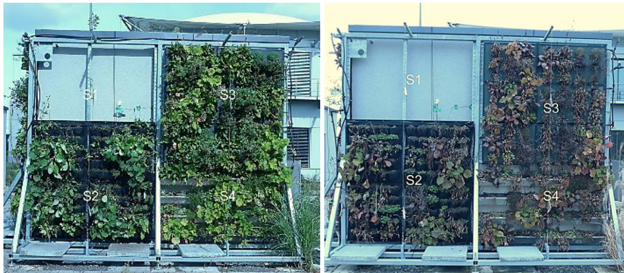
Fig. 7: South façade with three different LWS before the measurement period on September 20, 2023 (left) and near the end of the measurement period on February 2, 2024 (right).
