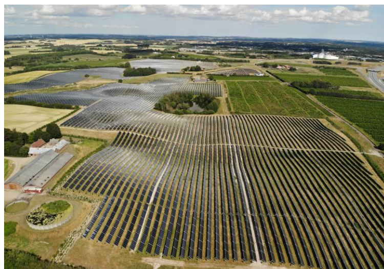
Fig. 1: Solar district heating plant in Silkeborg (156,694 m 2 )
