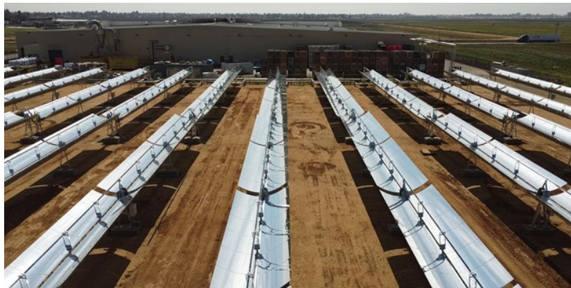
Figure 1. 2.3 MWth solar steam facility for almond pasteurization in Madera, CA [(Epp, 2022), Image credit: Sunvapor]
