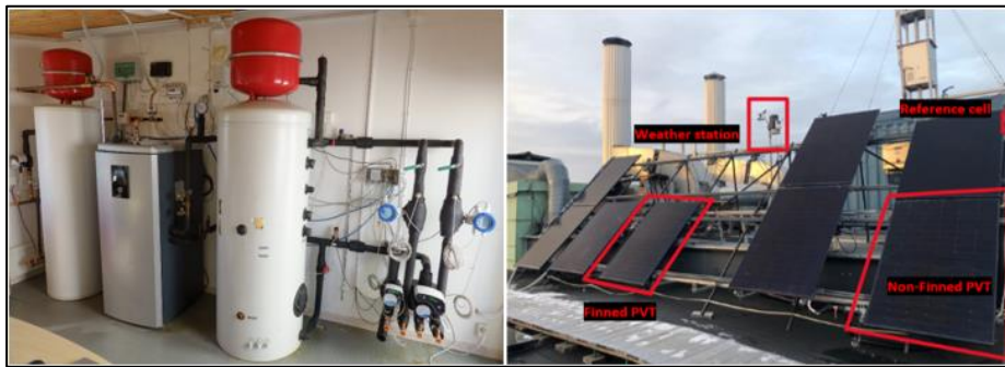
Fig. 1: Left) Mechanical room containing the HP and hot and cold storage tanks, as well as the circulation pumps and their monitoring system. Right) Test rig with the PVT collectors being tested.
