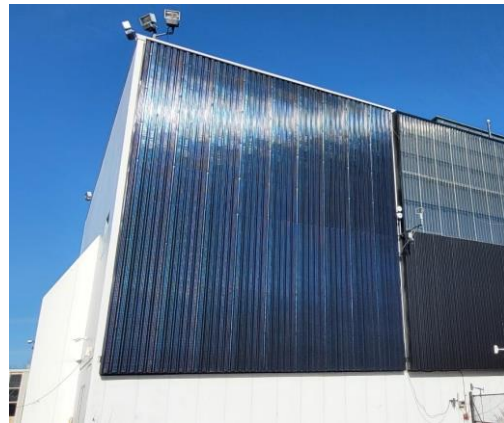
Fig. 4: Installed collectors. left: unglazed, selective surface model, right: two-stage black paint model.
