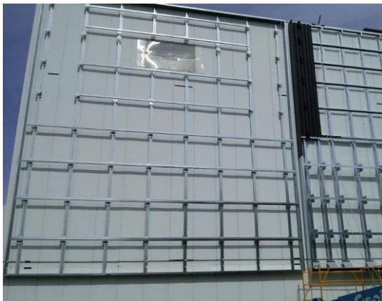
Fig. 3: Transpired solar air collectors under construction at the Canadian National Solar Test Facility.
