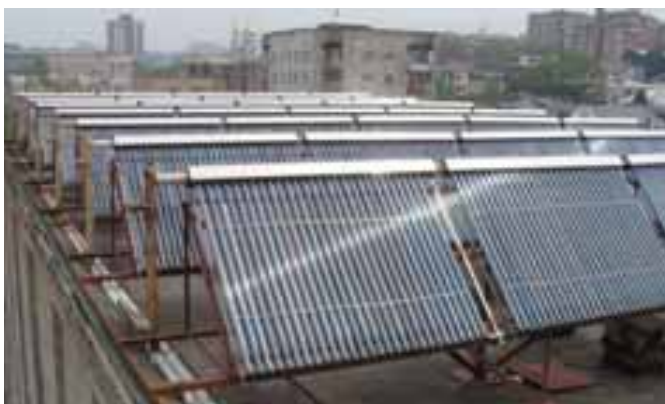
Fig. 1 - General view of the experimental SWHS, its solar collectors (roof of the Far Eastern Federal University, campus building)
