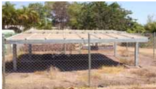
Fig. 1: The Outdoor Solar Facility for the 1.5 kWp CIGS system (ENER TSG200-GS2, Inverter: EnaSolar1.5KWGT-AUNZ)
