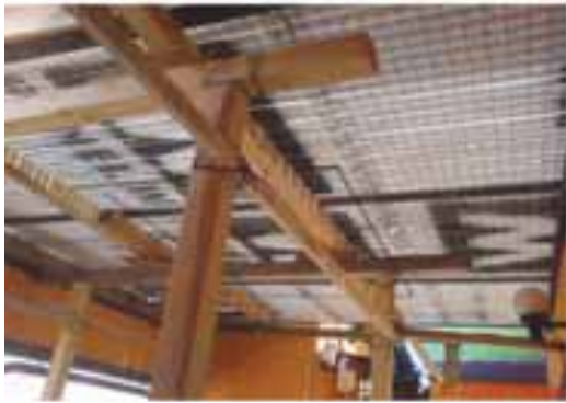
Cover construction process
