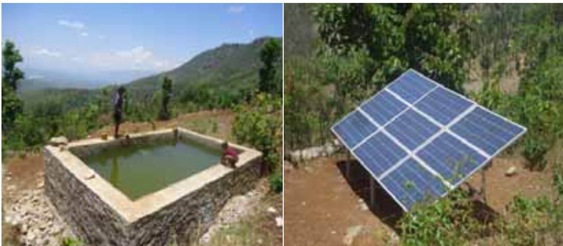
Figs. 11 & 12: PVWP system and water storage tank used for vegetable farming at Pokharikada, Surkhet, Nepal.
