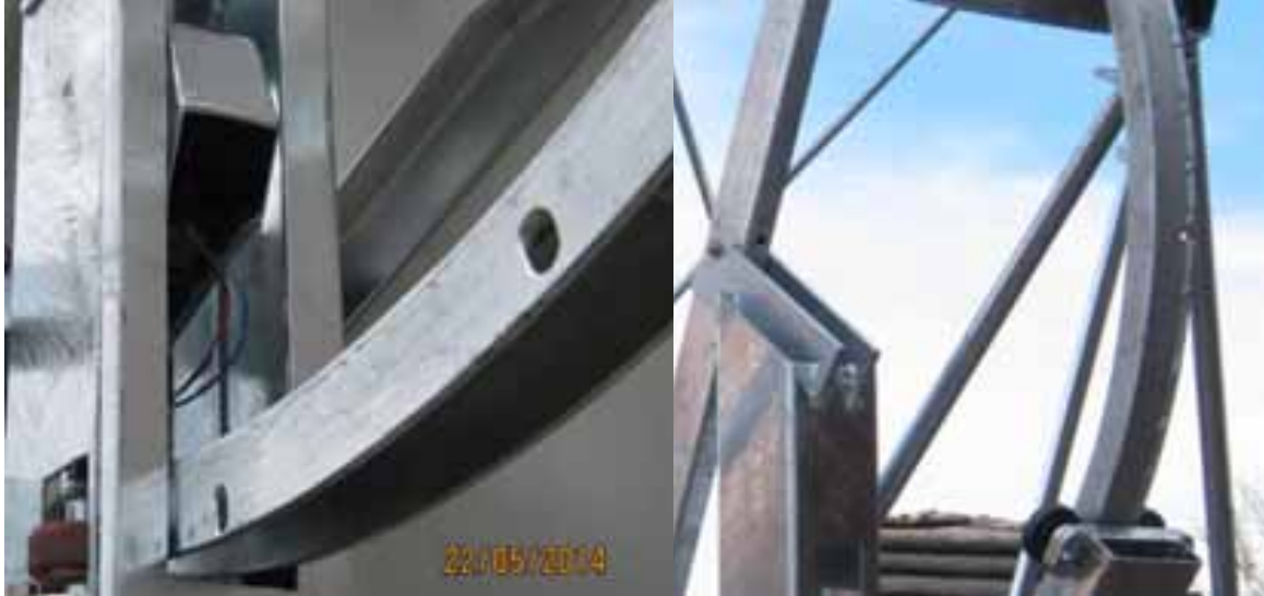
Fig. 12: “U”-profile of 1st rim (left); closed profile of 1st rim (right) for increased stiffness.
