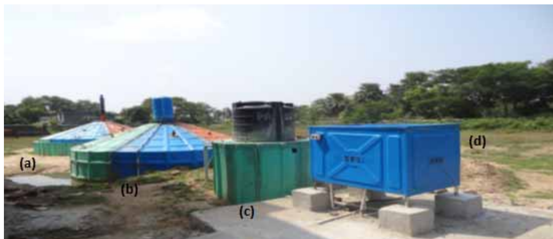
Fig. 2: Components of the AD system: gas chamber (a), main digester (b), predigester (c), chopper/grinder (d).
