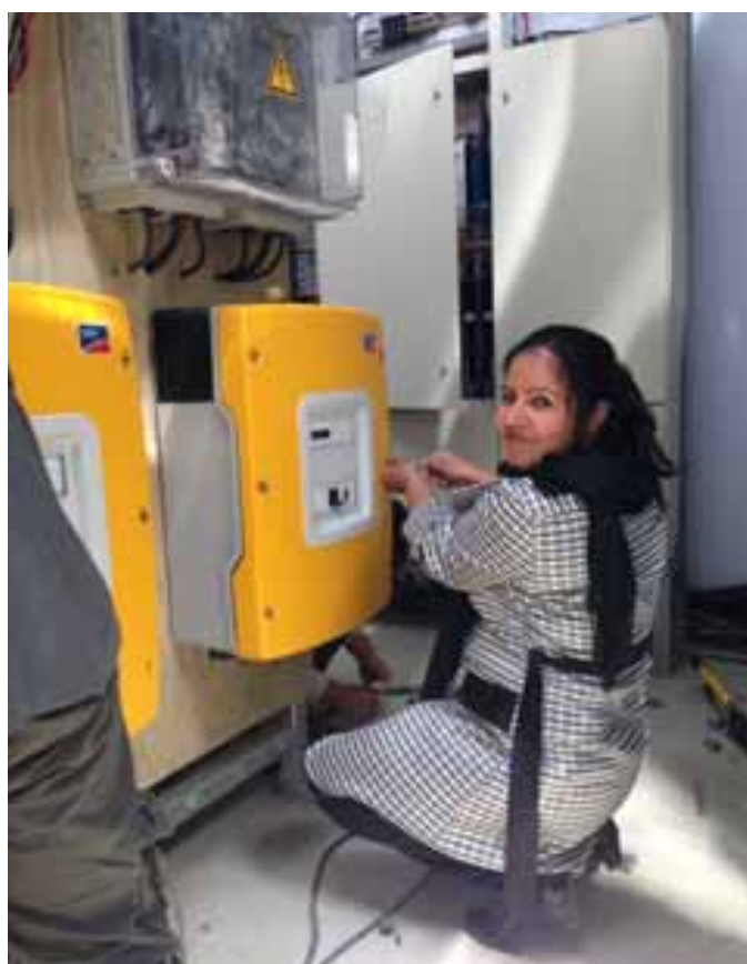
Fig. 6: SESI trained and utilized Afghan women technicians as part of the installation crew.
