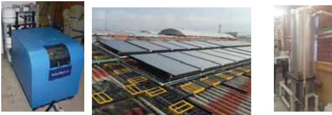
Figure 4. Installing components of solar cooling system
