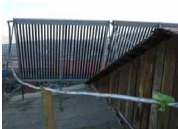
Fig. 3: Solar circuit pipe to return
