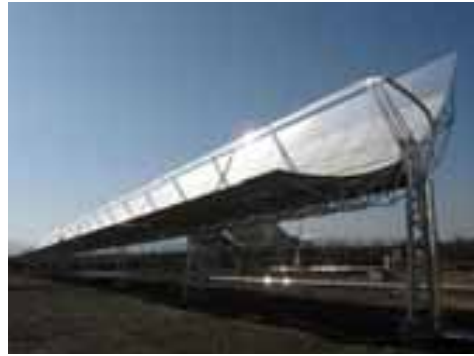
Fig. 1: Trough concentrator (The picture is from National solar thermal Union)
