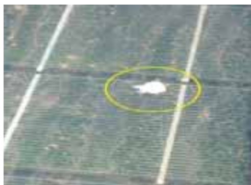
Fig. 6: Fauna droppings on the panels - 1 st August 2014
