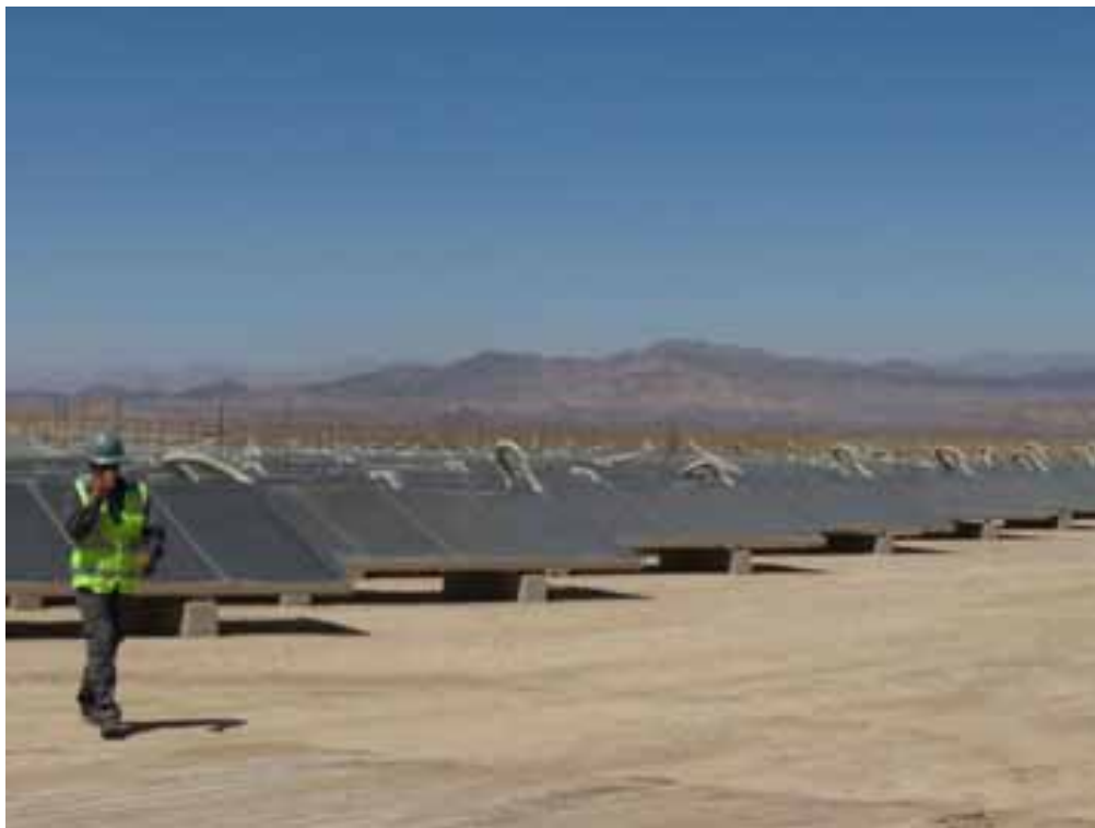
Fig. 5 Part of the flat plate collector field at “Pampa Elvira”. The tilt mechanisms can be seen
