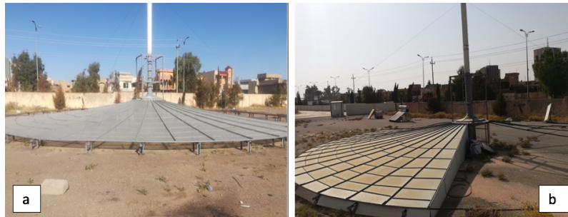
Figure 5: Showing the experimental rig when the collector was shape. (a) Front view of the rig showing the air inlet area (b) Side view showing a sealed side
