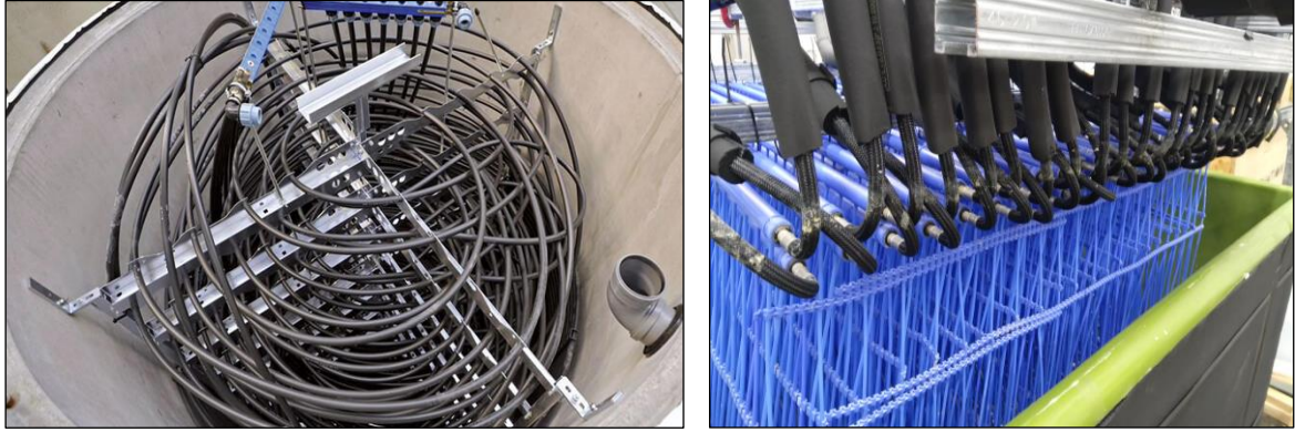
Fig. 1: (a) Cylindrical Ice storage with helical coil heat exchanger geometry from Viessmann Werke (on left) (b) Cuboidal Ice storage with U-type capillary mat heat exchanger from Clina (on right)
