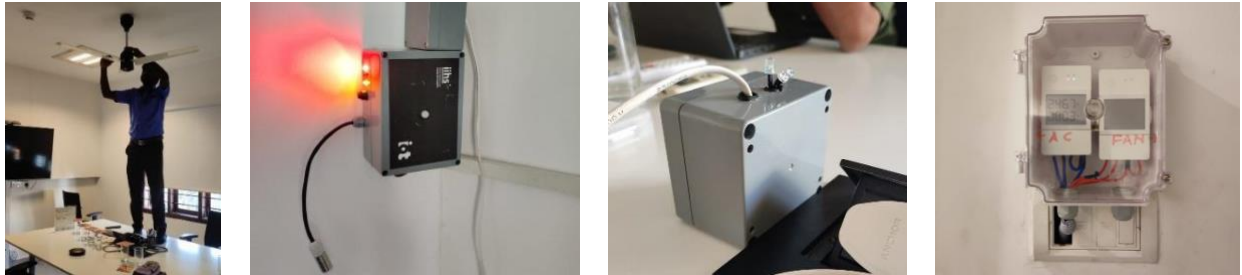
Figure 2. Images of the hardware installed in each room (a) BLDC ceiling fan, (b) IEQ box, (c) IR blaster, (d) energy meters.
