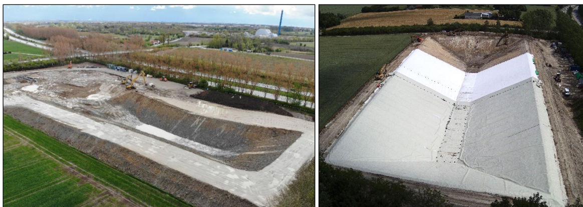
Fig. 1: Excavation (left) and liner installation (right).
