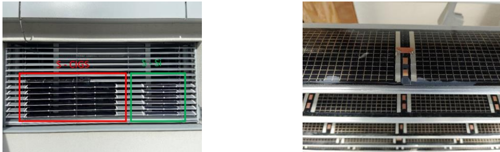
Fig. 7: Application of the PV-Modules on the Testbed (left) and detail of the S – CIGS Module (right)
