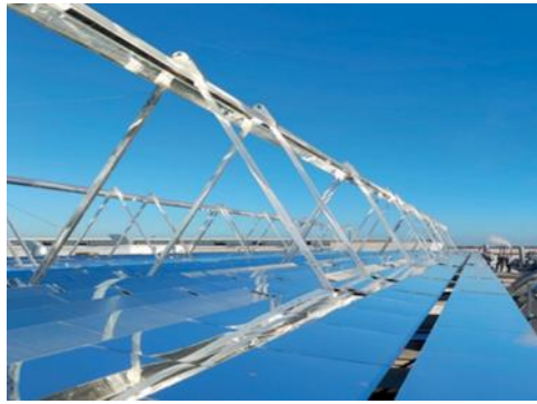
(a) Photograph of the Fresnel concentrator
