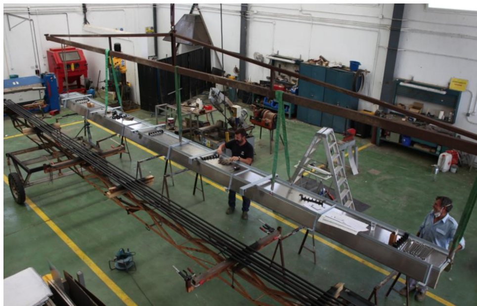
Figure 4: View of the LFC during the assembly of parts in the PSA workshop.
