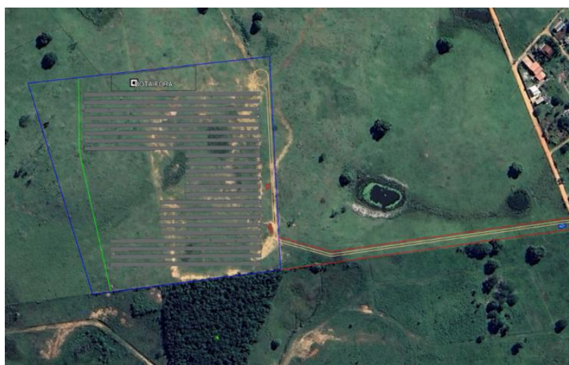
Figure 2: Location map of the photovoltaic power plant in Iguaba Grande, Rio de Janeiro, Brazil. Source: Google Earth.
