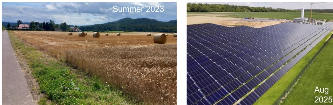
Figure 3: Construction site before the start of construction and after completion of the work.
