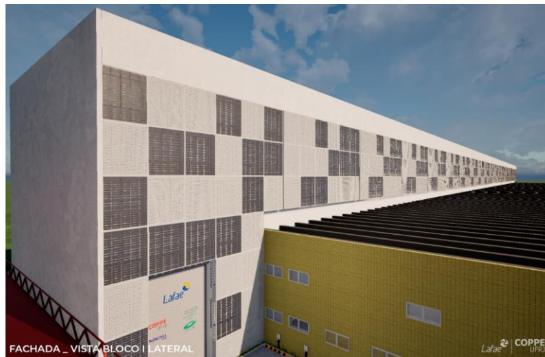
Figure 5: Side view of the façade of Block I, highlighting the distribution of photovoltaic modules along the vertical surface and their adaptation to the geometry of the building.
