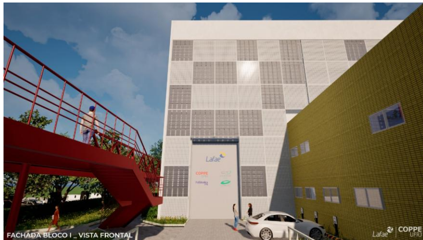
Figure 4: Front view of the façade of Block I with the integration of photovoltaic modules, showing the uniformity of the arrangement and the aesthetic compatibility with the architectural retrofit.
