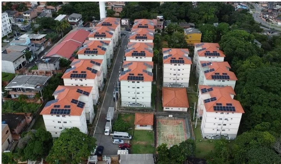
Figure 1: Plants installed in the Mané Dendê Condominium
