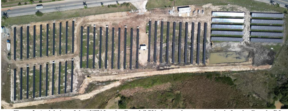
Figure 2: Aerial view of the “UFV Iguaba Grande” PV plant under construction in Iguaba Grande, RJ.
