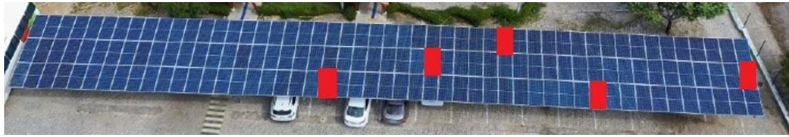
Figure 4: Monitoring layout of modules (Font: Author, 2025).
