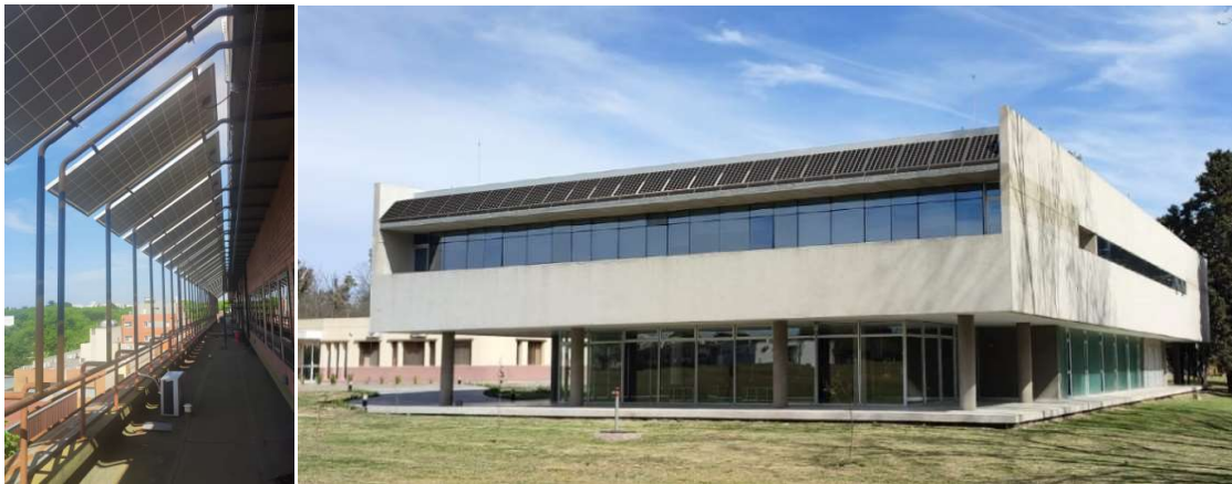
Figure 4: BIPV installations. A semitransparent pergola (left), and one forming the eaves of the building (right).
