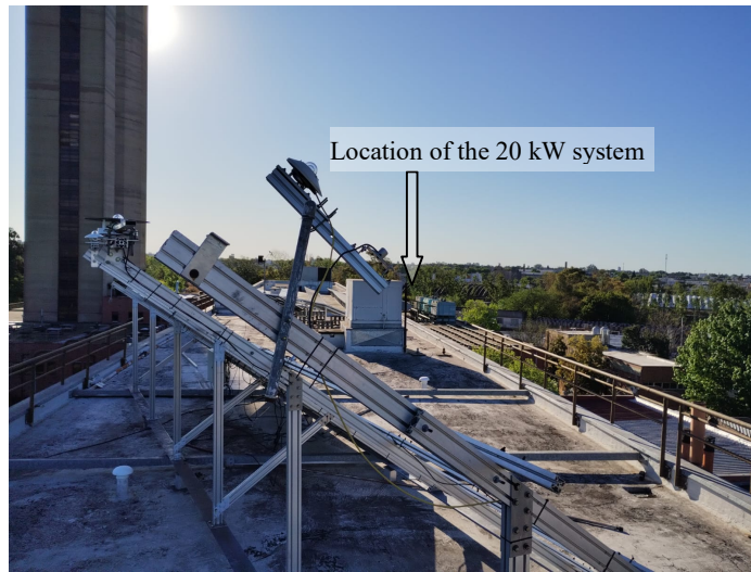
Figure 6: View of the radiometers bench under the shadow of TANDAR accelerator tower. Approximate location of the 20 kW system is indicated.
