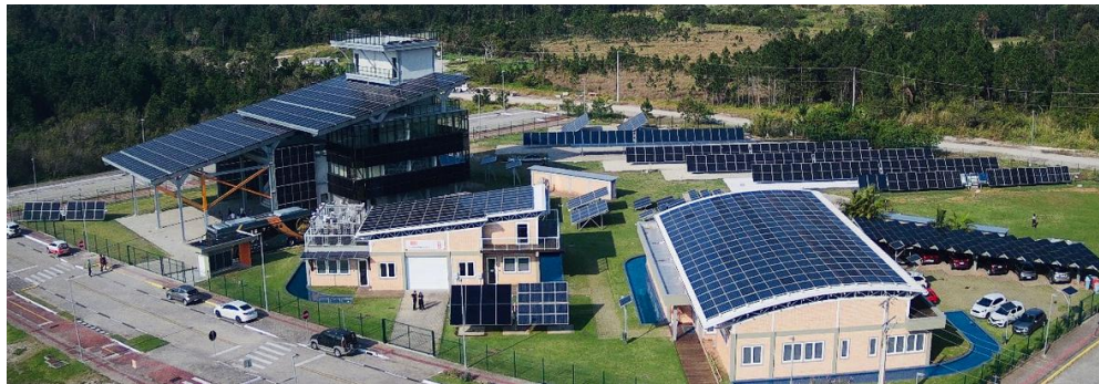
Fig. 2 – Buildings A, B and C of the Laboratory
