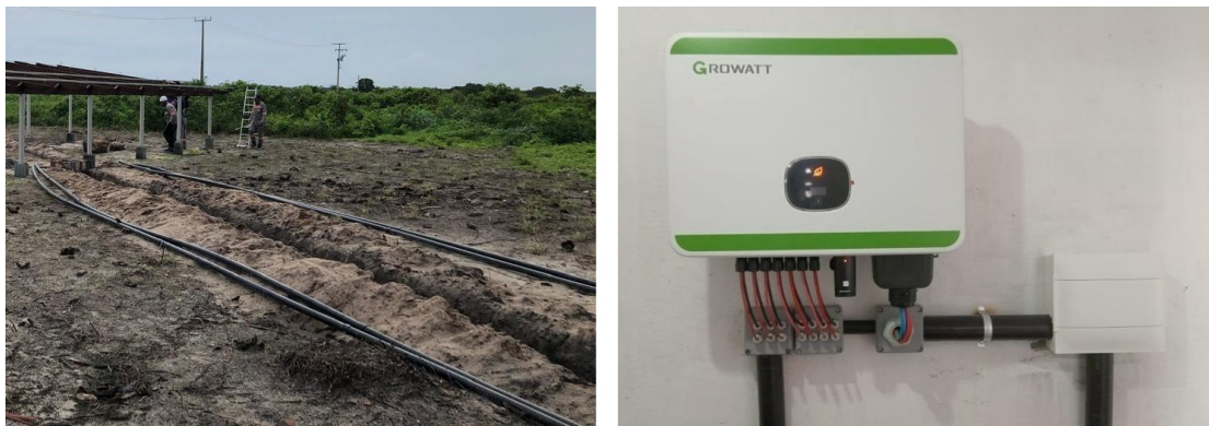
Fig. 2: Installation of 2-inch polymer conduits (left) and DC/AC solar inverter (right) [Authors]
