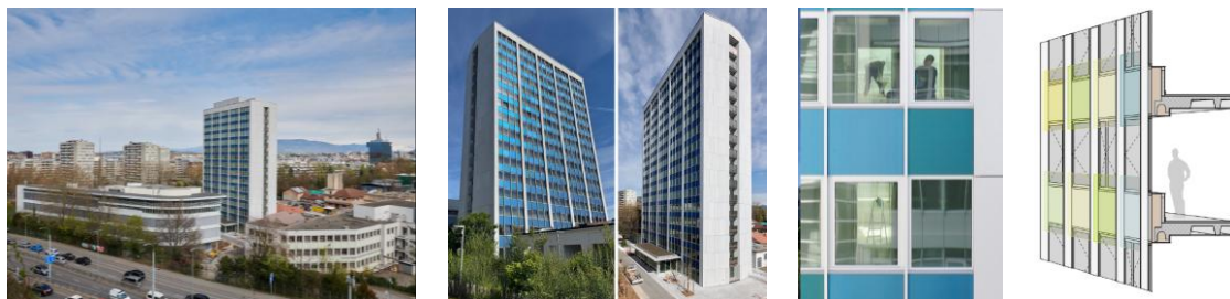
Figure 7 Firmenich Tower within urban context, view, elevation and section of façade-integrated BIPV systems (Photos Baud&Fruh)
