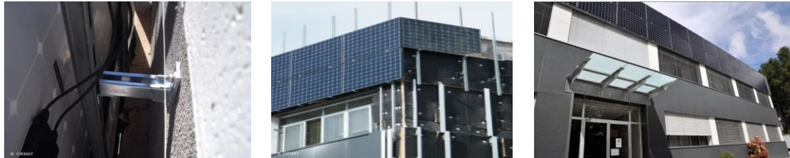
Figure 3 CIEMAT Building in Spain with the details of BIPV ventilated façade (Photo by N.Martín Chivelet © CIEMAT)
