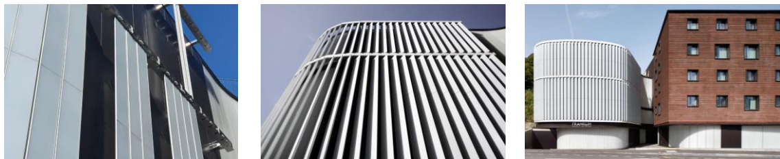
Figure 6 Franklin University Switzerland (FUS) and white rotating photovoltaic louvers (Photo by Leo Torri)
