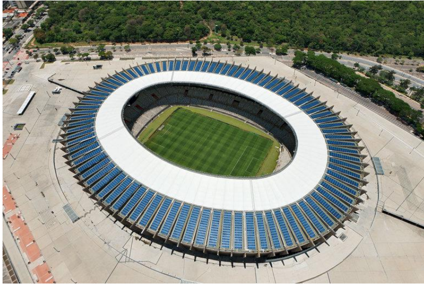
Figure 1: Aerial view of the Mineirão Stadium photovoltaic (PV) system, featuring 5,910 solar modules spanning 9,500 m 2 of the stadium's roof in Belo Horizonte, Brazil.
