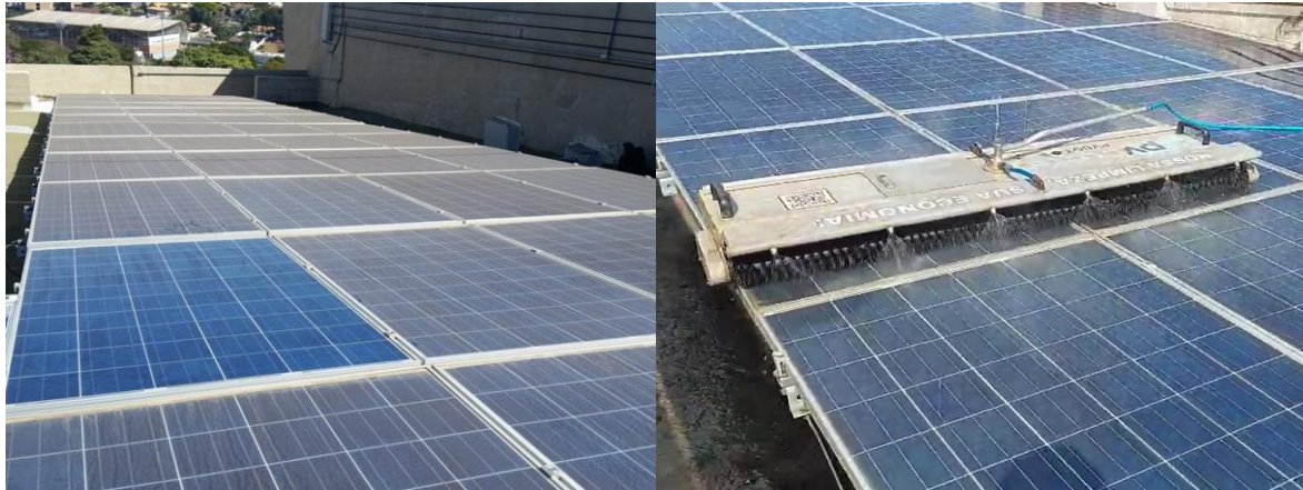
Figure 12: Left – Water access constraints complicate manual cleaning at the top of Mineirão Stadium. Right – Robotic cleaning systems now enhance efficiency and quality.
