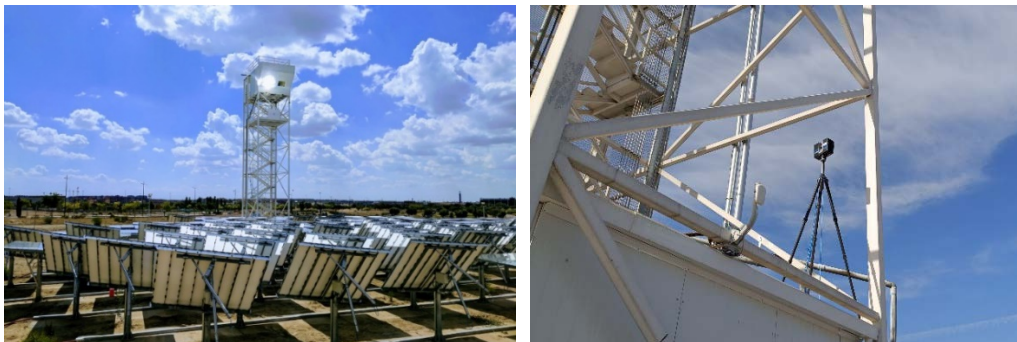
Fig. 1: a) IMDEA's solar field in operation; and b) Terrestrial laser scanner from FARO.
