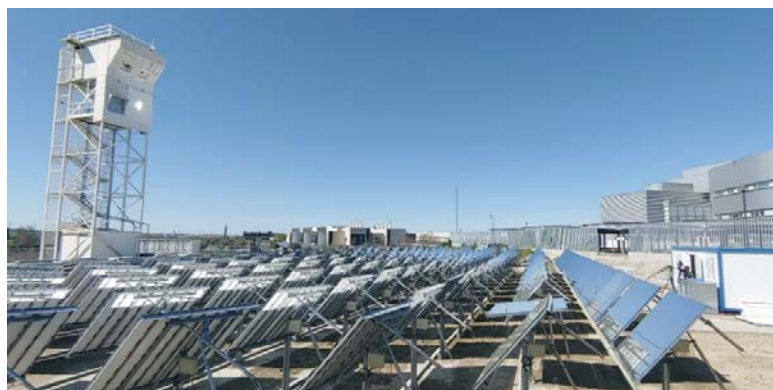
Fig. 1: Solar field at IMDEA Energy with the field on stand-by and one heliostat pointing to the target at the tower. The camera setup is located on the right side of the photograph near the control room.
