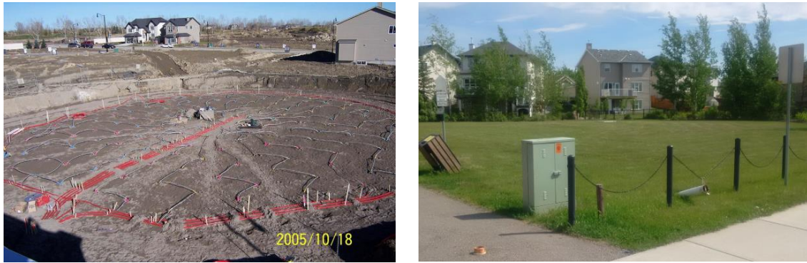
Fig. 3: Borehole field under construction and currently, as a landscaped park
